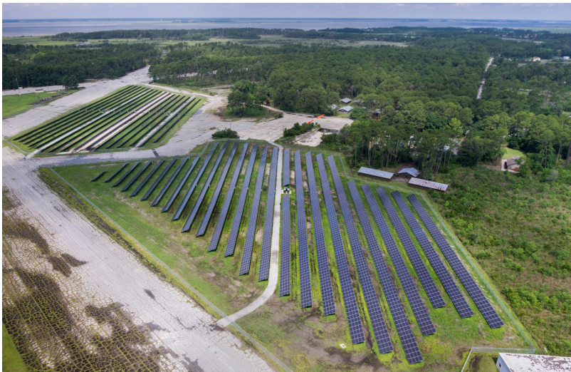
➤ The 5.7 megawatt on-site solar photovoltaic array, placed on the old Parris Island air strip, covers 50 acres. Photo courtesy of Ameresco.
