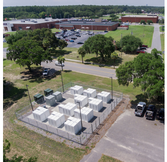
➤ The 4 megawatt/8 megawatt-hour Tesla battery energy storage system at Parris Island can monitor peak loads and discharge to the base grid as needed. Photo courtesy of Ameresco.
